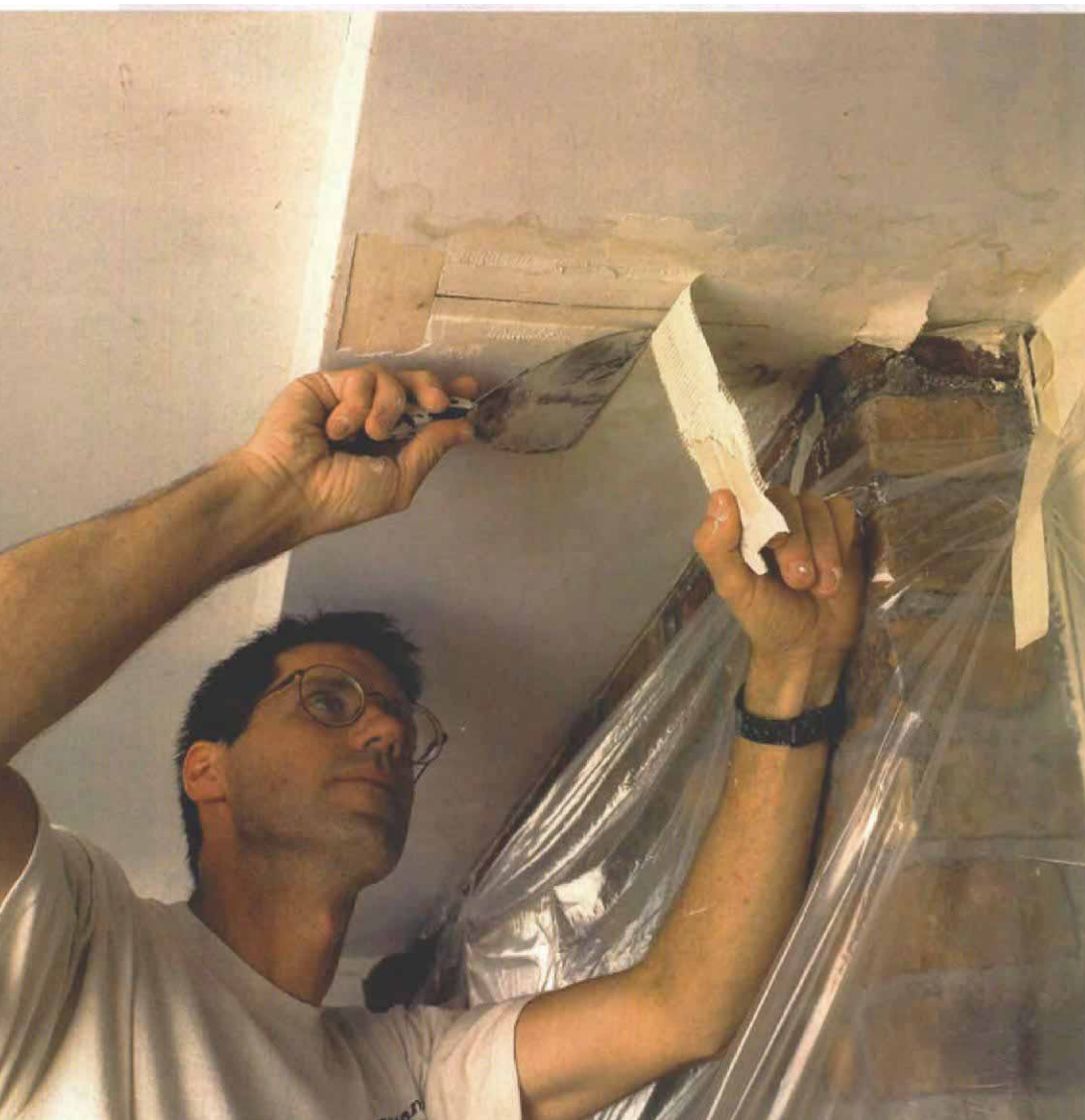
Bevel edges of the wall opening , then cut a matching piece and bevel its edges.
